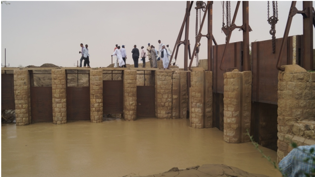
Photo 3: Side of the field visit: main regulator on Khor Abu Habil (on the right) and the gates diverting water to the main canal feeding cultivated areas in El Rahad
