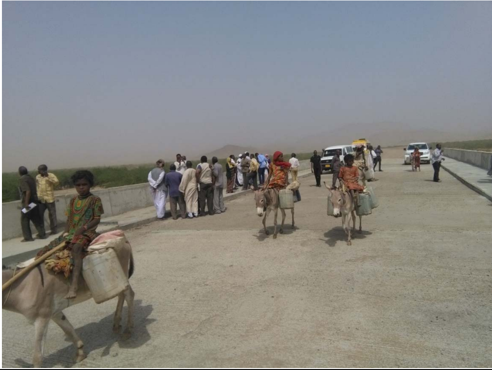
Photo 8: The bridge crossing Khor Baraka
